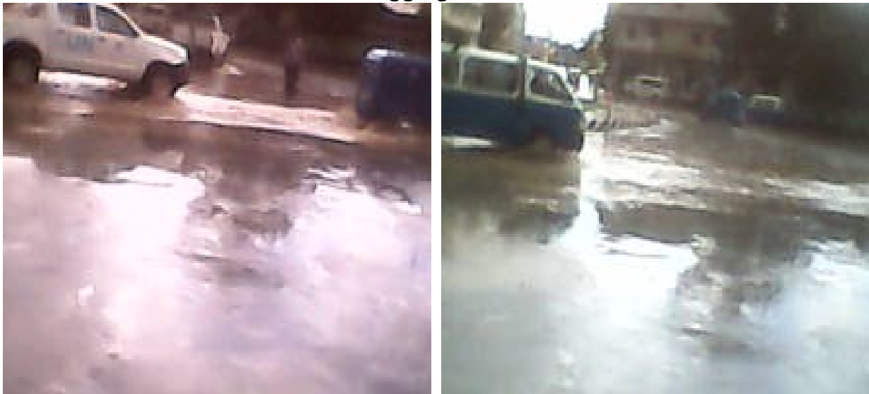
Figure 55 Water Logging Area of Bazar Roundabout (Source: Own)
