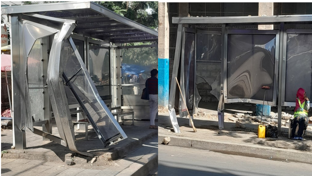
Figure 4.5: Damaged Bus Stops (at Mekanisa and Mexico Lideta) Source: Photograph taken by the Author (October, 2022)
