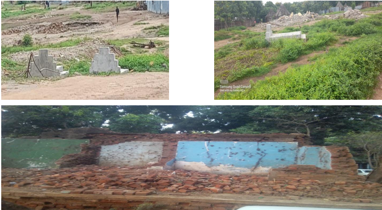
Figure 4.19: Tomb within residential area demolished
