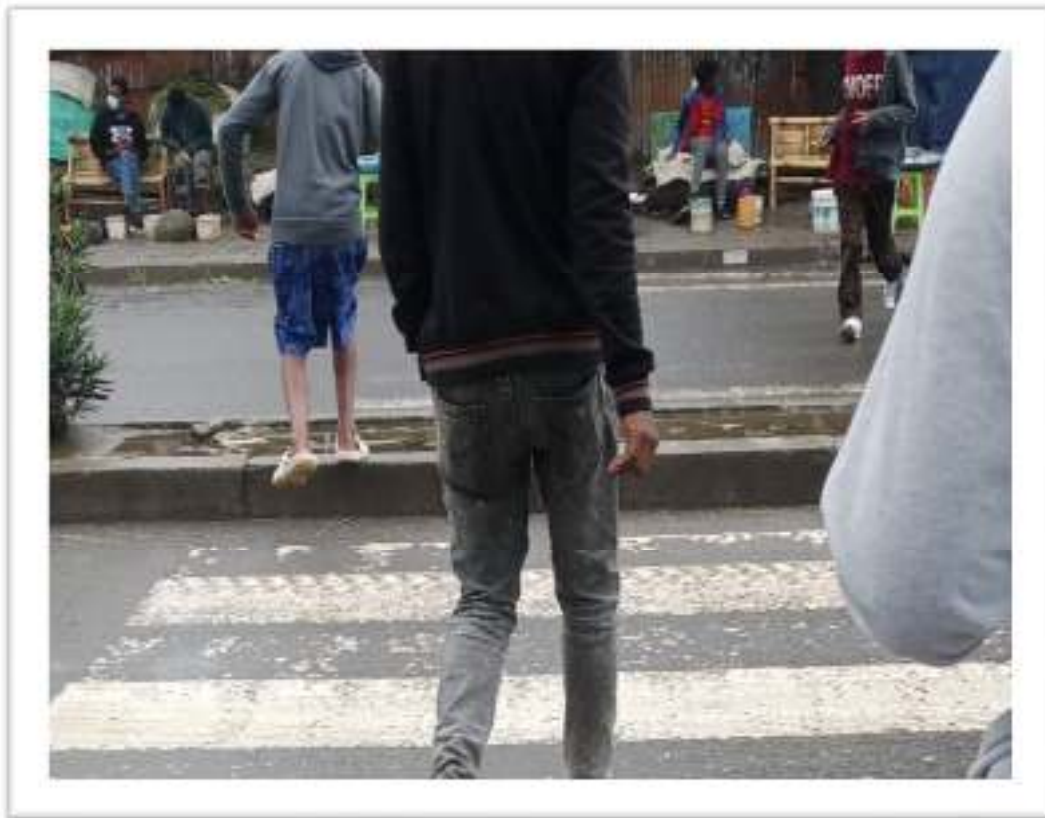
Picture 4.6.1.7 Median without ramp and narrow without proper structure in Mikael
