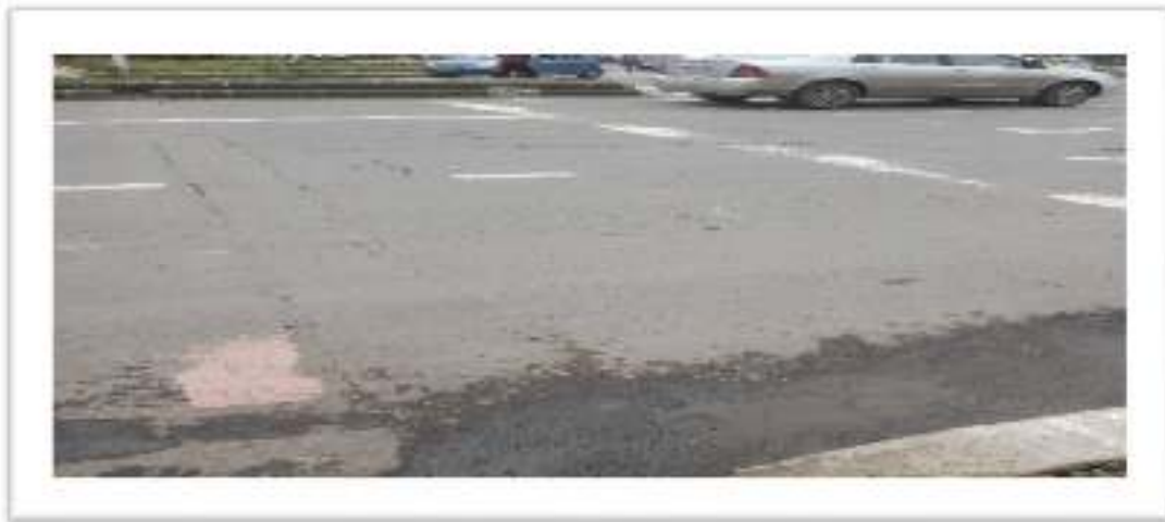
Picture 4.6.1.10 Unparallelled crossing in tikur ambesa
