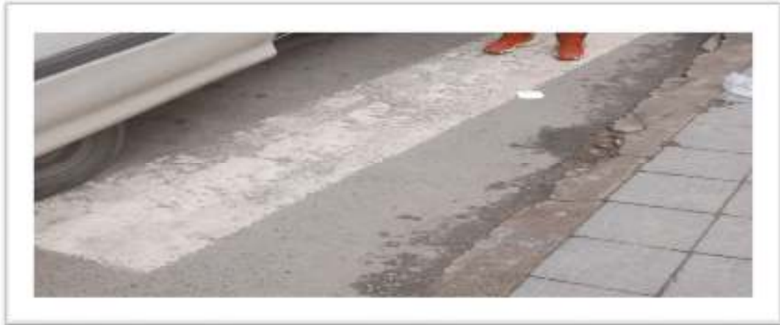
Picture 4.6.1.11 Uncomfortable ramp structure in mexico and taxi using zebra crossing
