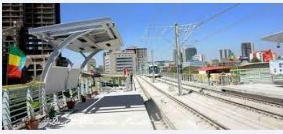
Figure 2.4 Light rail station facility to show extreme weather condition resistance.
