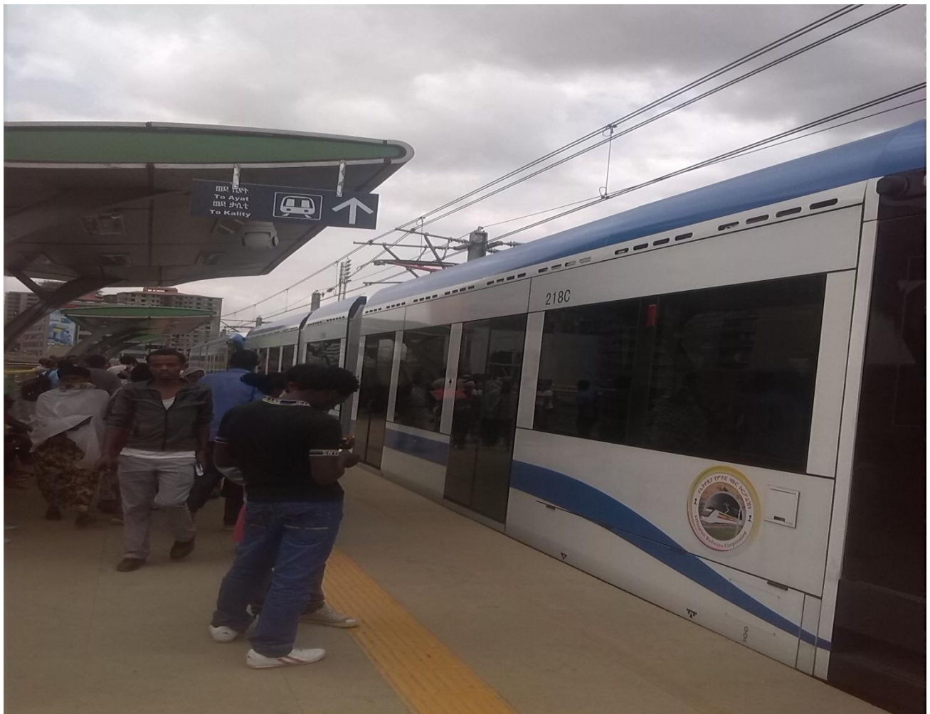
Figure 4.2 Stadium Station of AALRT the place both south- north rail meet west- east line which is common station for both line.
