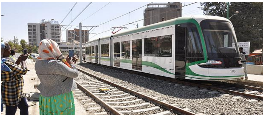
Figure 4.1 Light rail transit track at grade crossing and operation.
