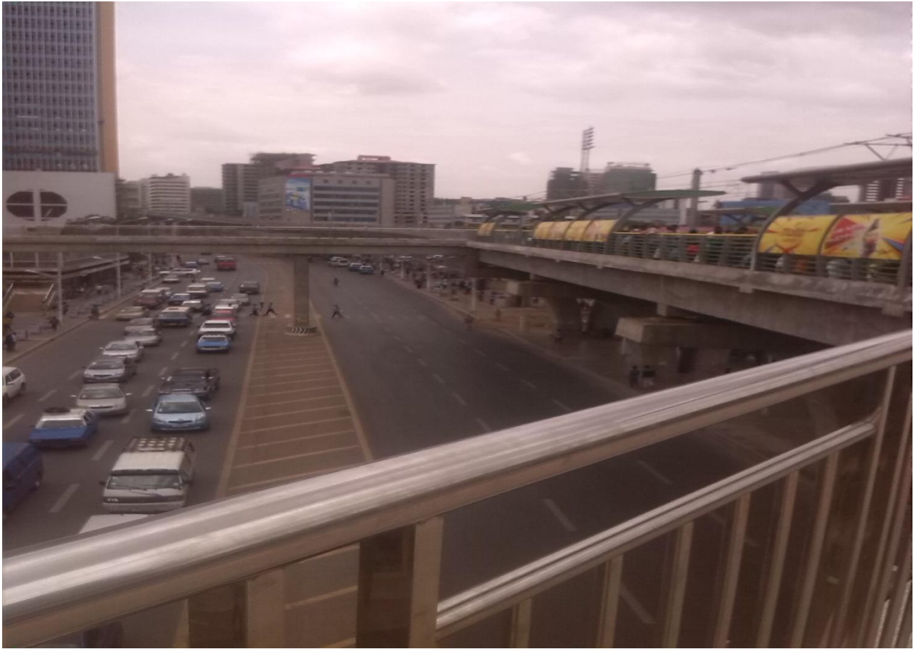
Figure 4.3 Access provided for elevated stadium station of AALRT
