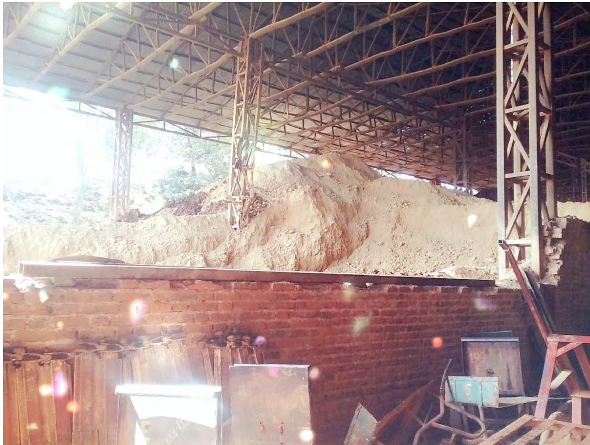
Picture B-1 Stock piled raw materials at Ethio Bricks
