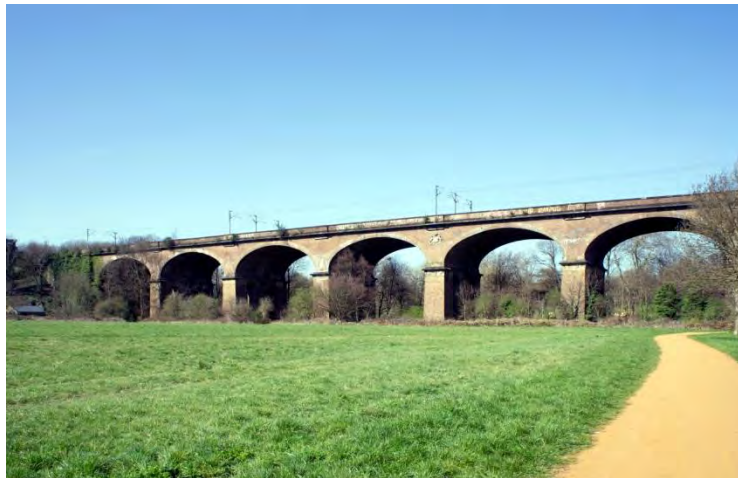
Figure 2-1: Han well railway viaduct, a brick arch structure [10]
