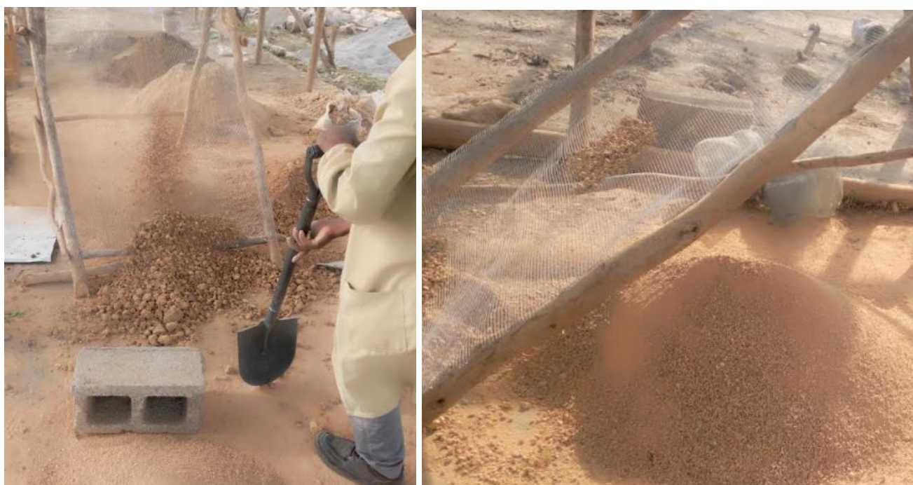
Figure3.1: Pulverization and screening of soil by simple manual technique
