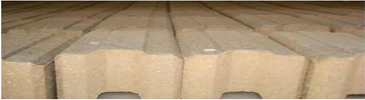
Figure2.3: Typical Interlocking CSEB Blocks Produced in STVC
