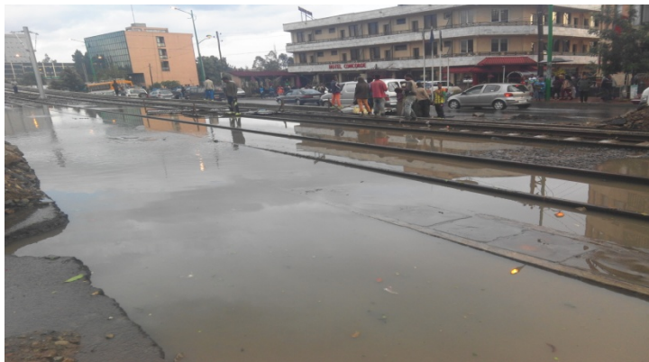
Picture no. 3 Flood event near Gotera
