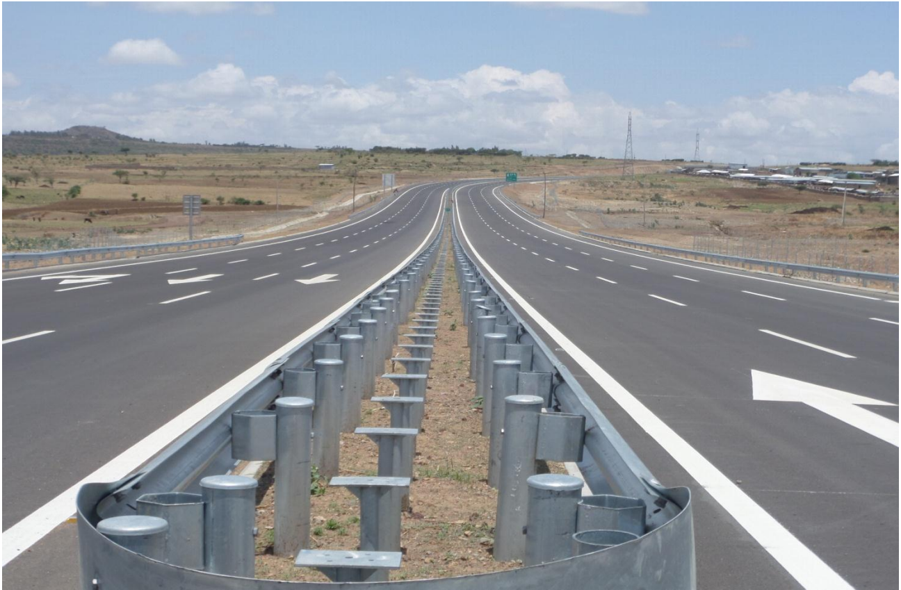
Fig. 3: Newly Built Addis – Adama Expressway Section (Semi-Manual System) [34]
