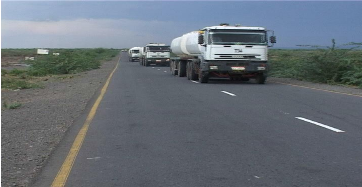
Fig.7: Typical section of the road corridor [on the rural area of the segment]
