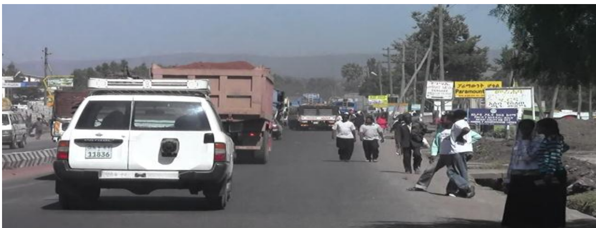
Figure 18: Existing Akaki –Kality road that does not have walkway for pedestrian and are functioning as single lane
