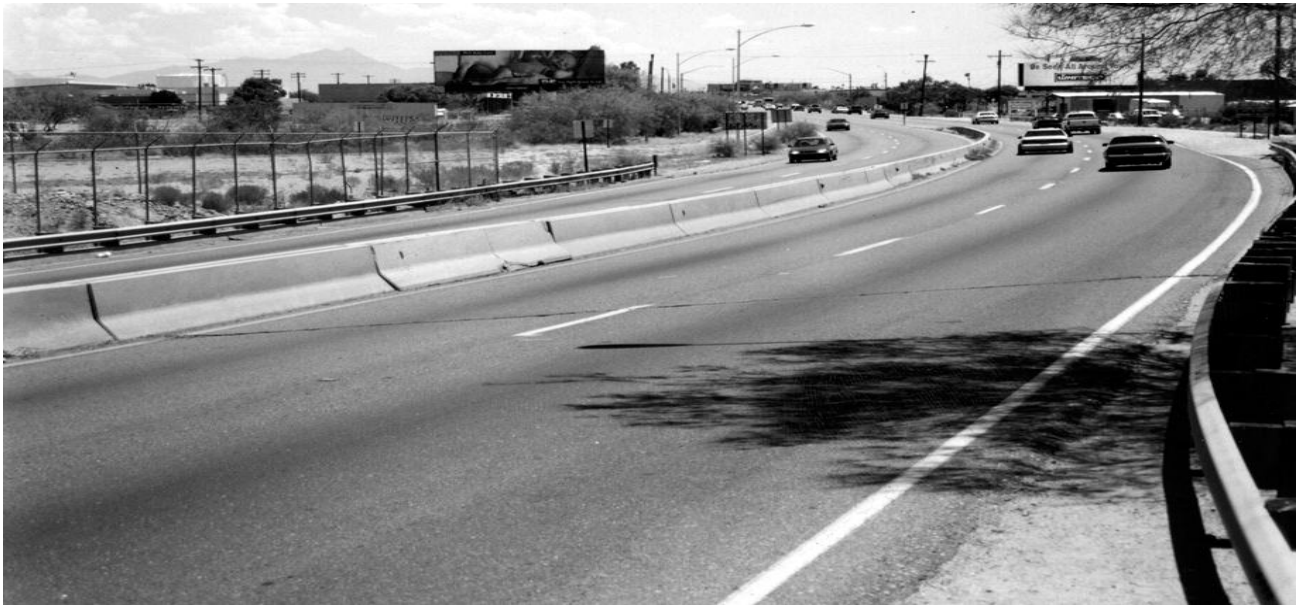
Fig. 8: Typical Divided Multilane Highway in a Suburban Environment
