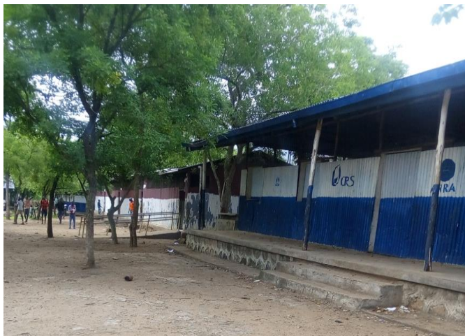
Figure 28: Classrooms and offices in Number 4 school
