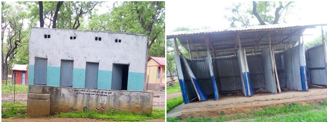
Figure 34: Toilet rooms in Number 2 School
