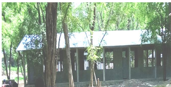
Figure 12: Classrooms under construction in Number 1 School
