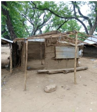
Figure 13: the image of roofless houses
