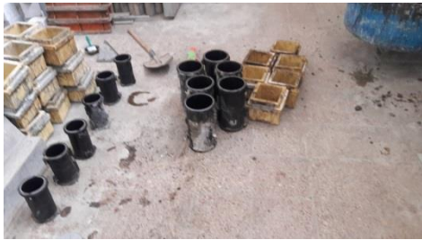
Oiling and preparing molds
