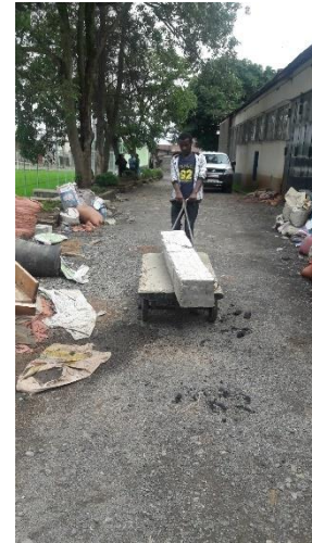
Depositing tested beam
