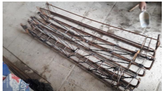
Figure 7: Preparation of concrete and reinforcement beam
