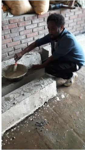
Painting and preparing experimental beams
