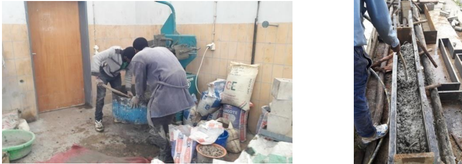
Figure 8: Mixing and casting
