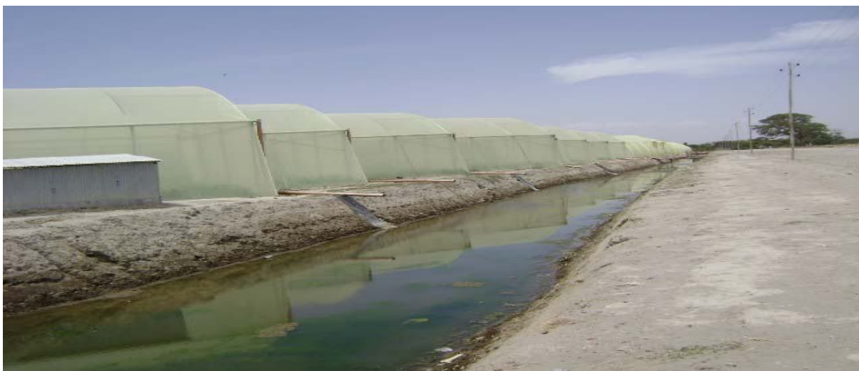
Figure 2-1: Direct effluent discharge to the lake
