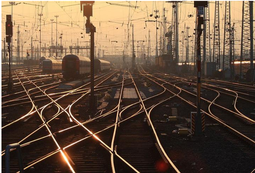
Figure 2-1: Turnouts at Frankfurt main central train station in Germany (Source: Wikipedia Commons)
