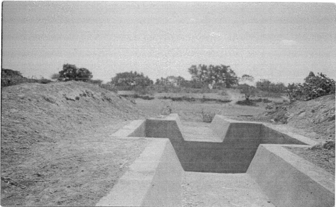
Figure 4: Pond constructed in Hurufa lola in 2006 by PSNP Public work participants
