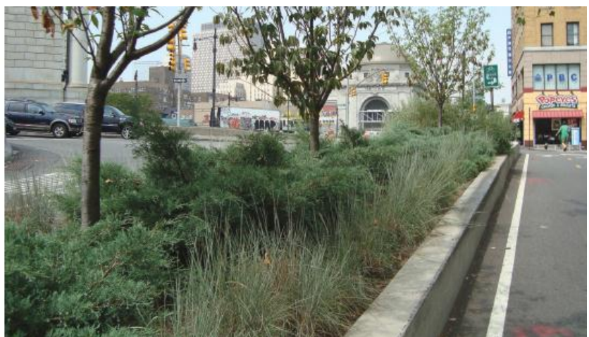
Picture 12: Planted raised median. (Source: SDM)
