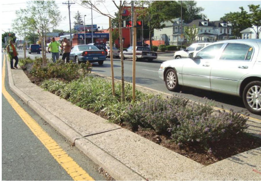
Picture 9: Curb-height median with plantings set back from the curb to allow easier maintenance (Source: SDM)
