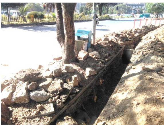
Picture 32: Trench cut through the main root system of street trees. (Source - Author)
