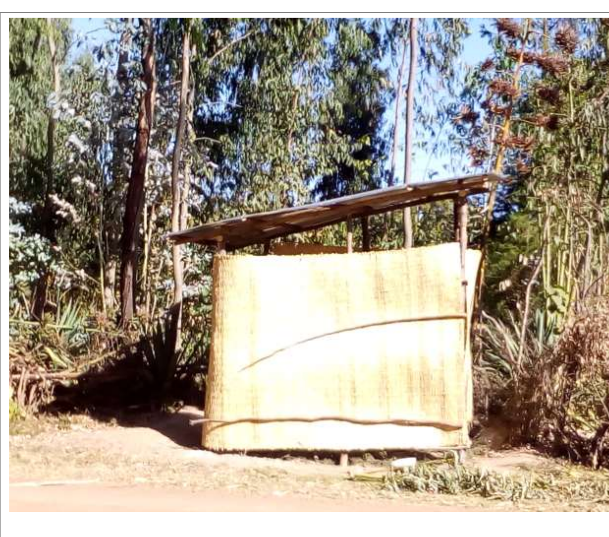
D) Public toilet in Ambicho
