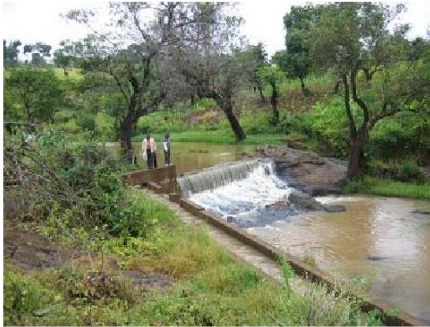
Figure 2.0.2: Example of an intake of a MHPP [8]
