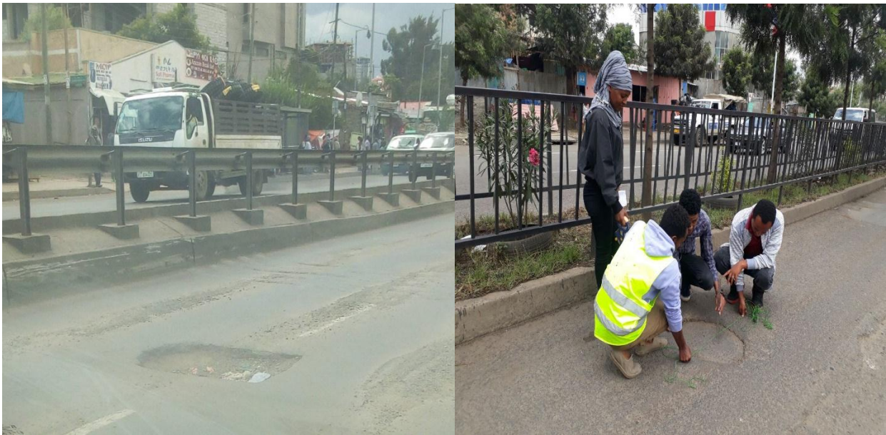
Mekanisa Abo to bridge road segment site condition
