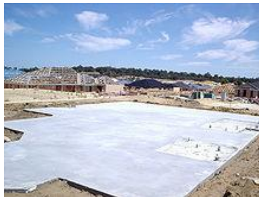
Figure 1:- Slab-on-ground/Slab-on-grade foundation
