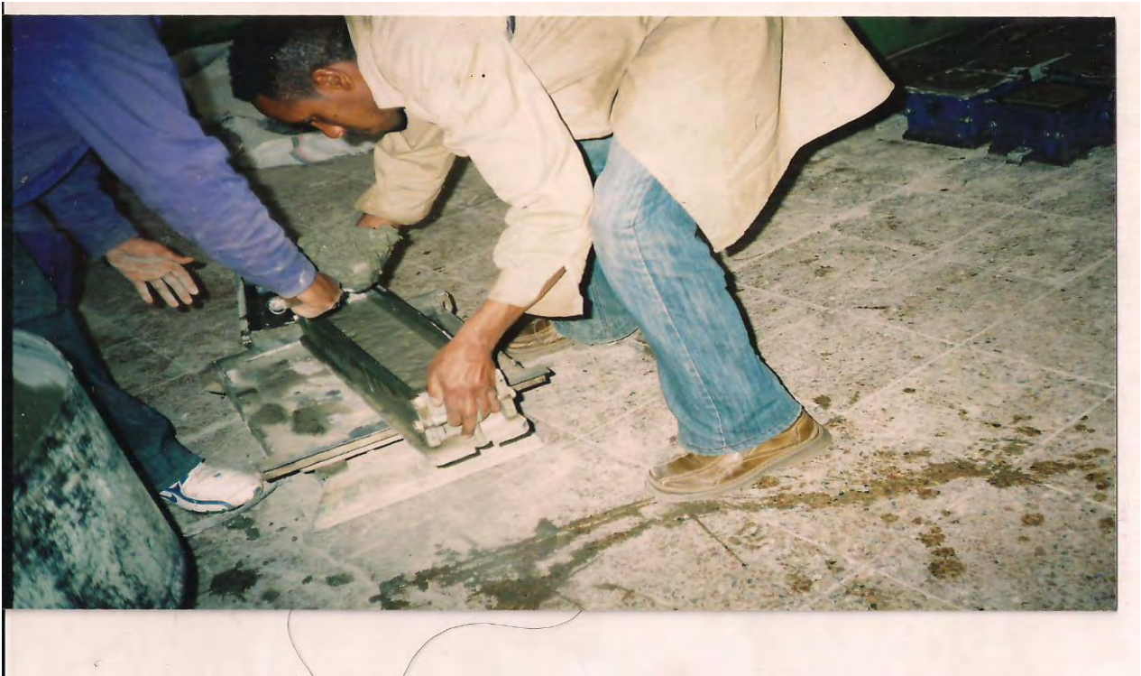
Photo 5: Placing of concrete into mold
