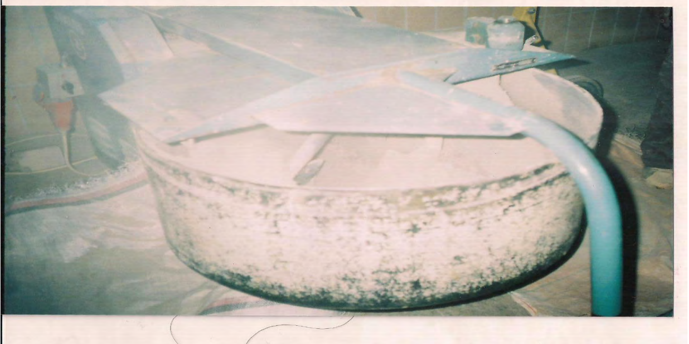
Photo 3: Mixing of concrete
