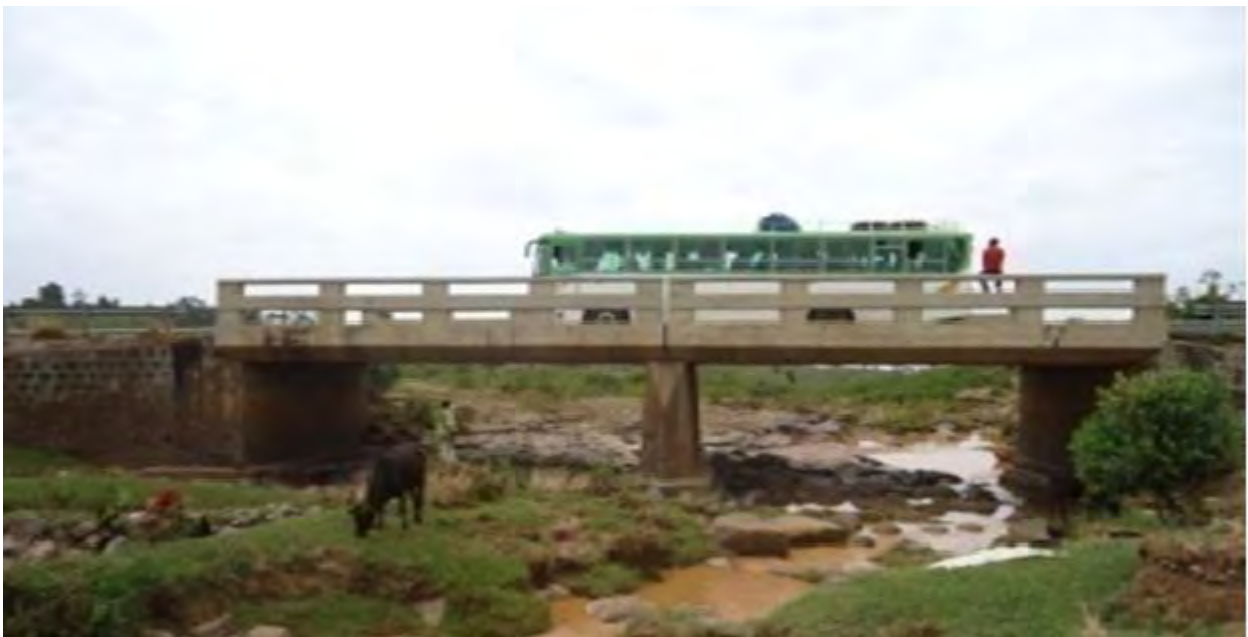
Figure 5.8 Previous bridge at chainage 47+100
