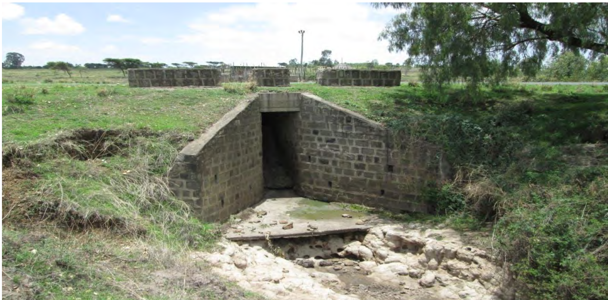
Figure 5.2 Existing culvert at chainage 81+430
