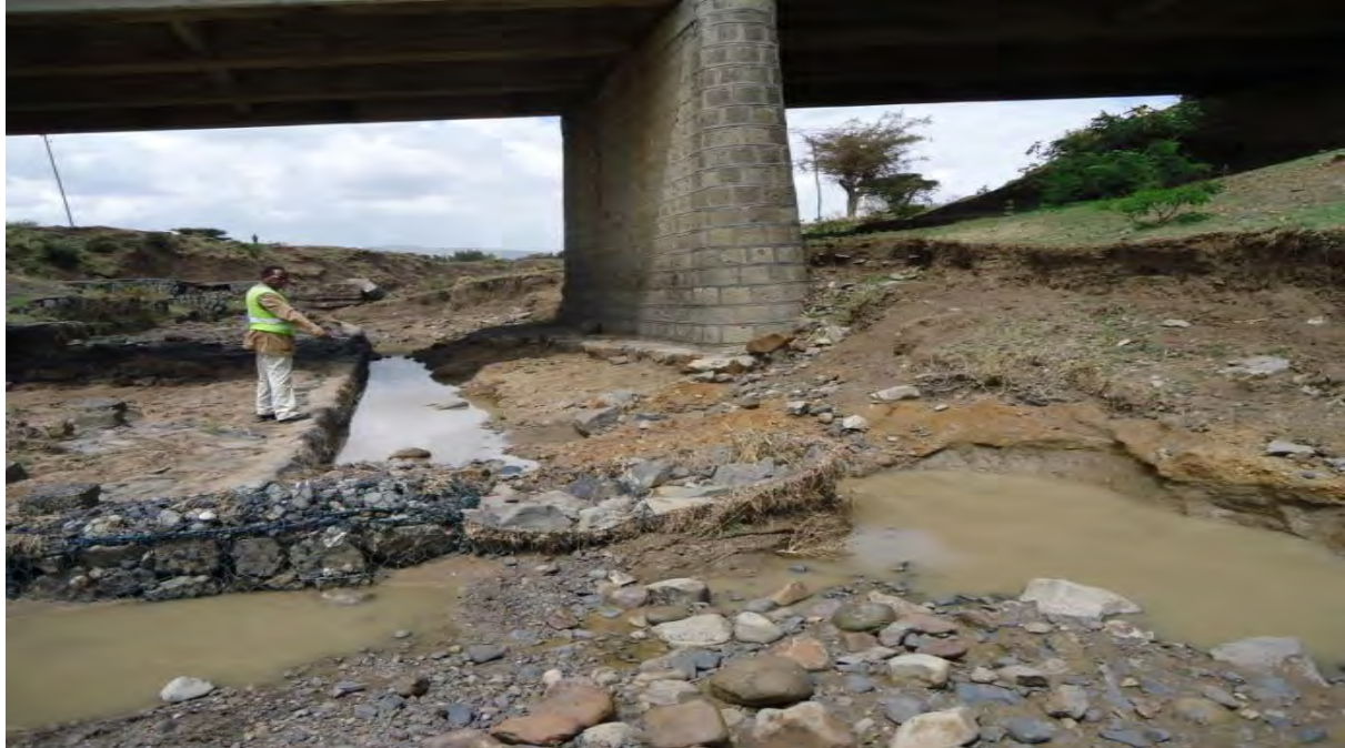
Figure 2.1 Typical Scour of Bridge at Pier
