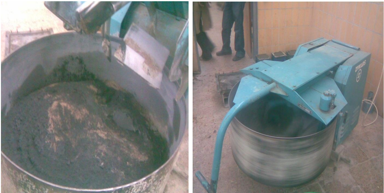
Photo 11. Concrete ingredients to be mixed (left) and being mixed (right)
