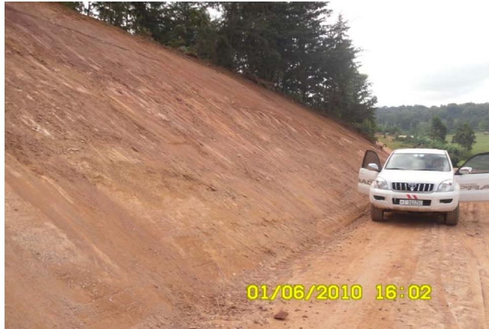
Plate 4.2 Typical sub-grade soils (Residual) in the road project (km 121+000, RHS)
