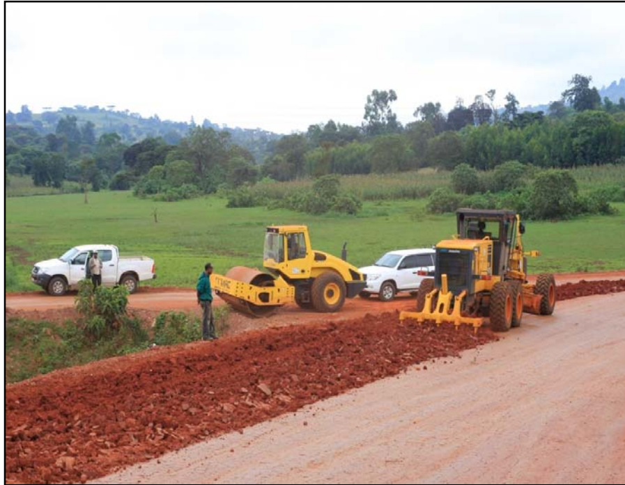
Plate 3.1 Partial view of the land use patterns (km 156 + 900), Photo September 2010
