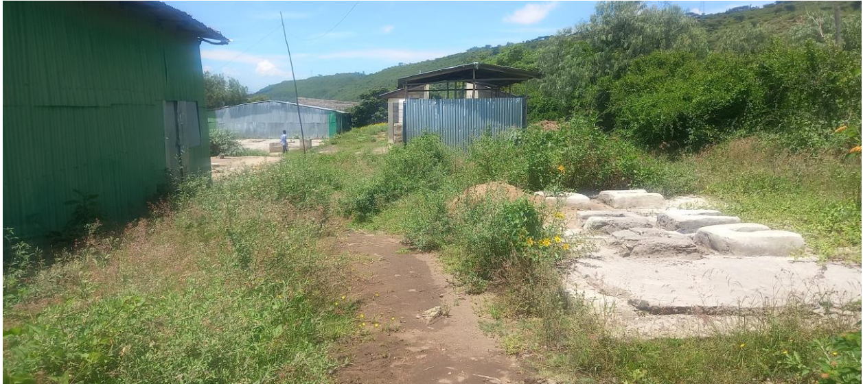
Figure 2: A toilet at Sena Seba School. Photograph taken by Mustefa Defo (May 02, 2024)
