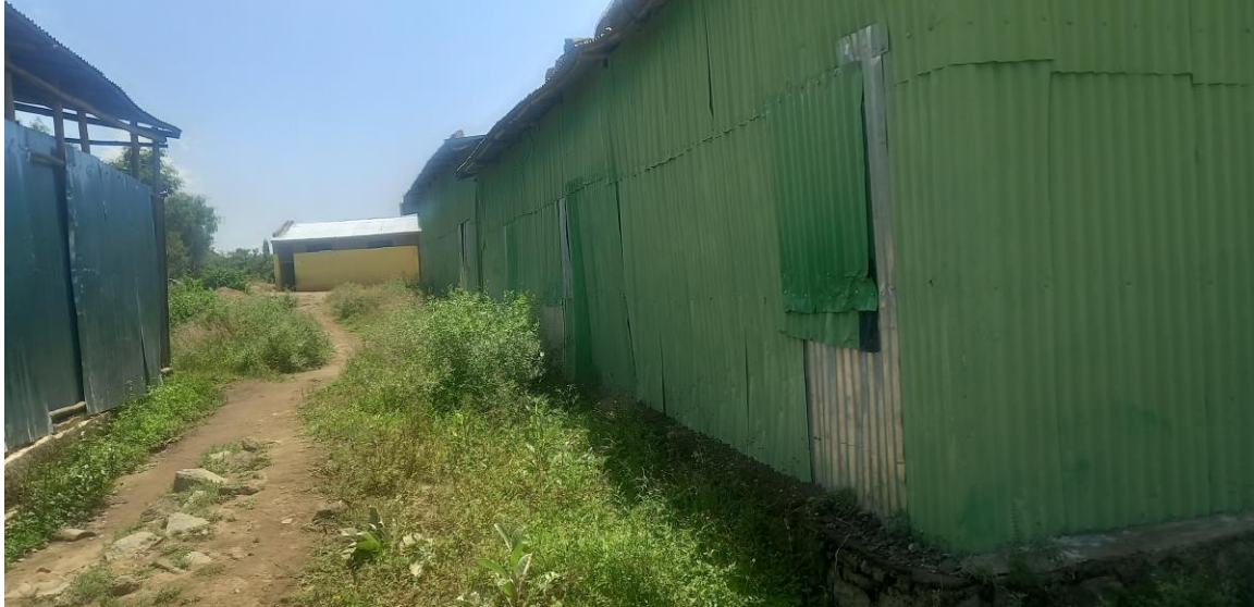
Figure 3: Class rooms made up of iron sheets. Photograph taken by Mustefa Defo (May 02 2024)
