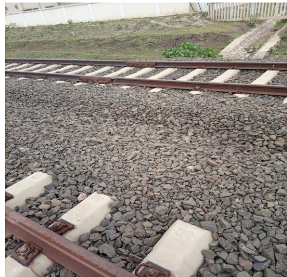
good ballast on straight line (non-critical)
