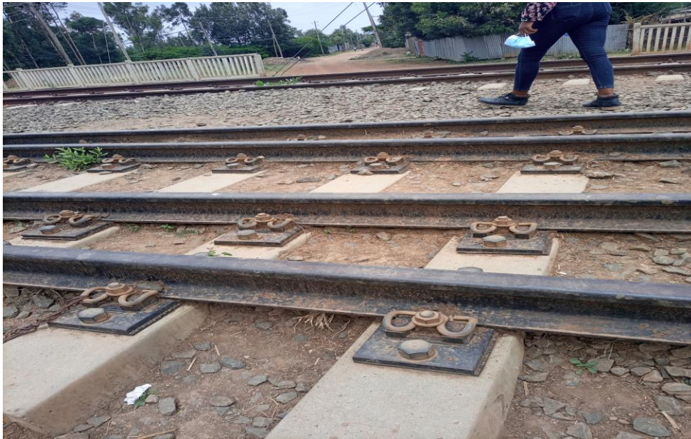
Figure 9. Deteriorated ballast(Sebeta)
