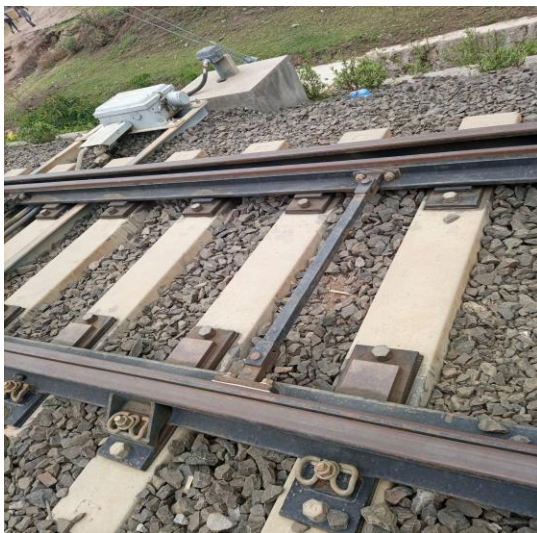
Figure 8. Ballast around turnouts and transitions(Furi,Indode) (fouling)
