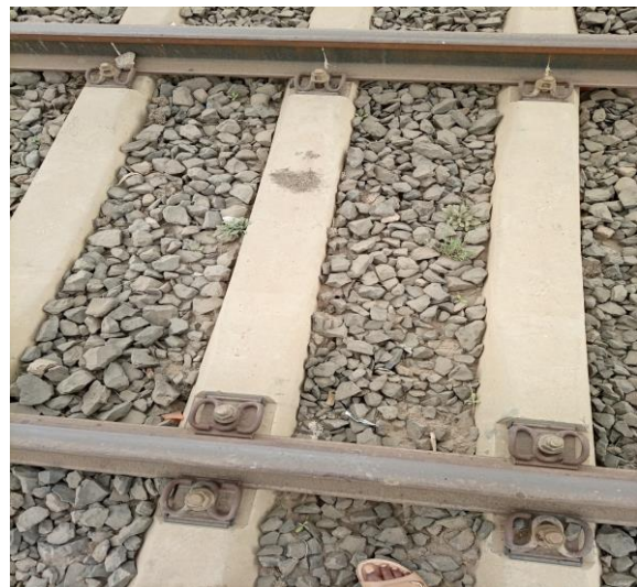
Figure 8. Ballast around turnouts and transitions(Furi,Indode) (fouling)
