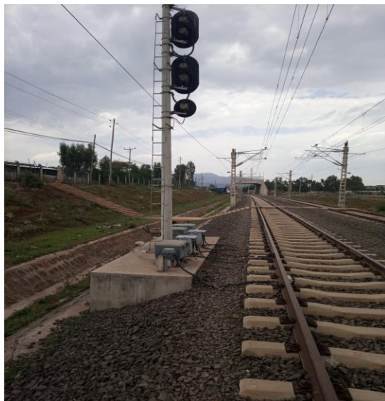
good ballast on straight line (non-critical)
