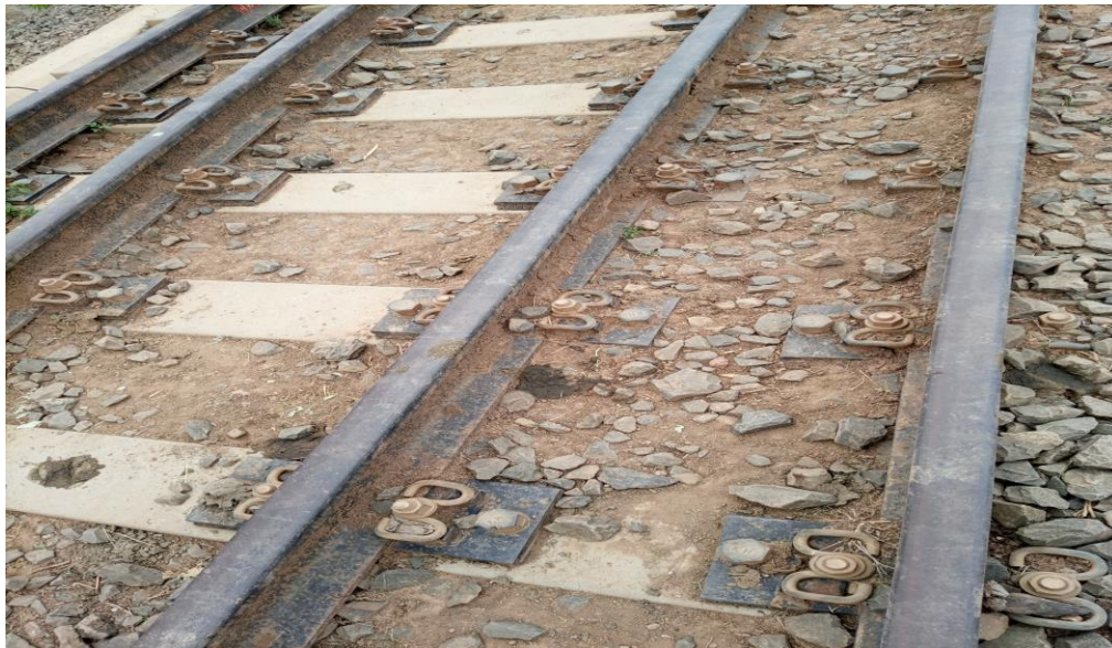
Figure 7. Fouled track ballast around undesigned crossings(Sebeta)
