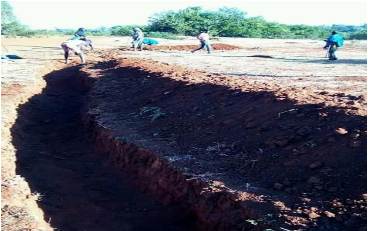
Figure 4: Soil bund /soil check dam in Enashenfalen kebele, photo from field observation
