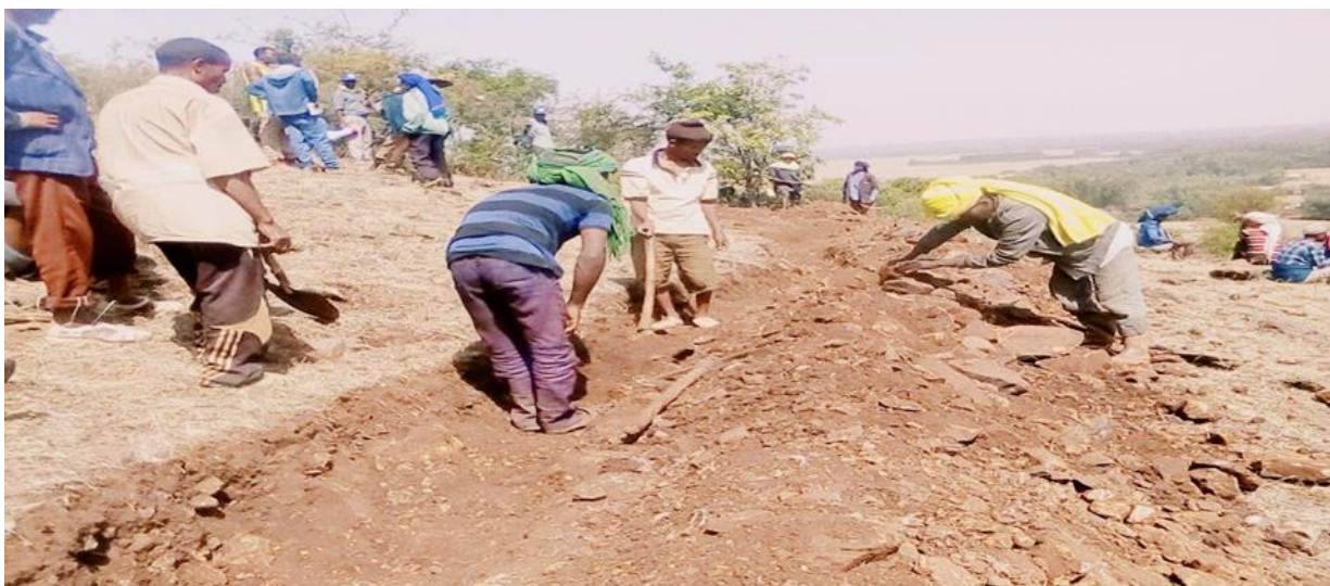
Figure 3. Stone –faced soil bound practices in Abromenor kebele, photo from filed observation.
