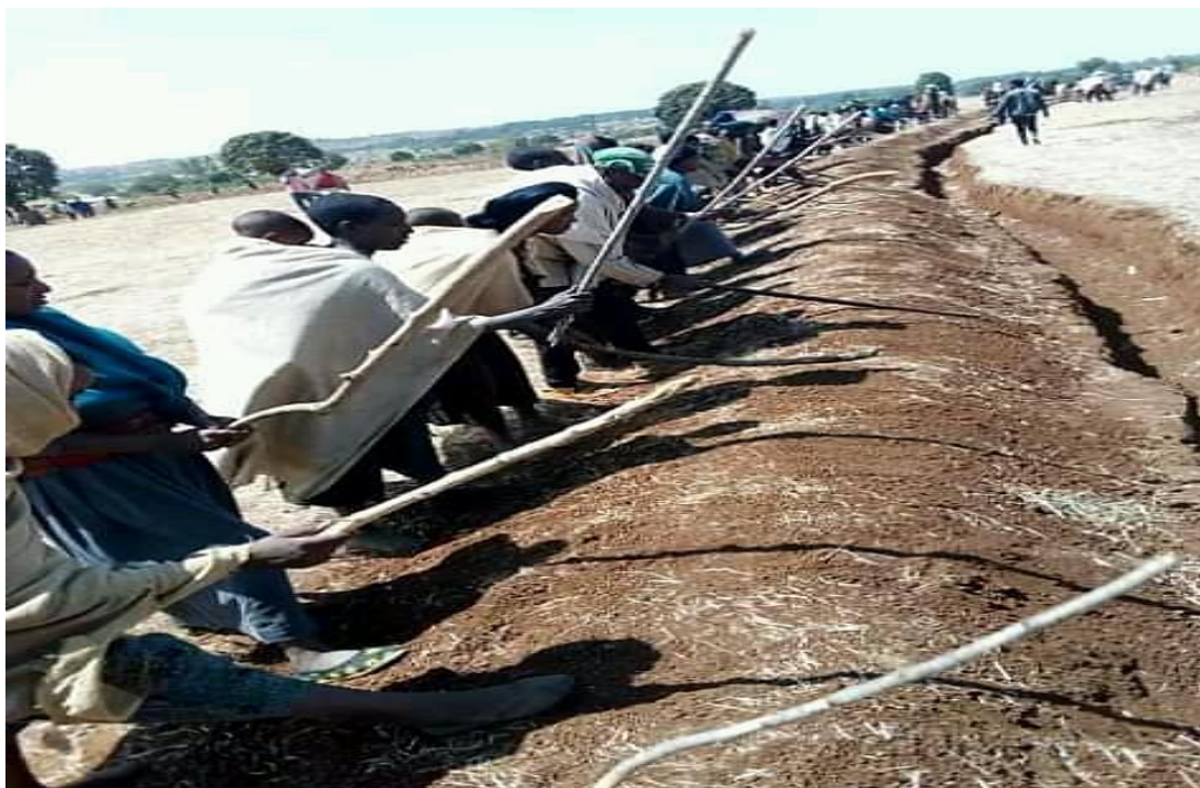
Figure 5: Fanya - Juu soil bounds with functioning drainage ditches in Enashenfalen kebele, photo from field observation
