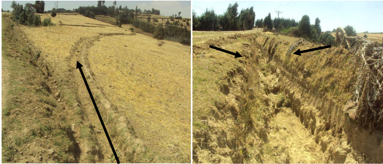
Figure 10: cut off drain (left) and Waterway (right).
