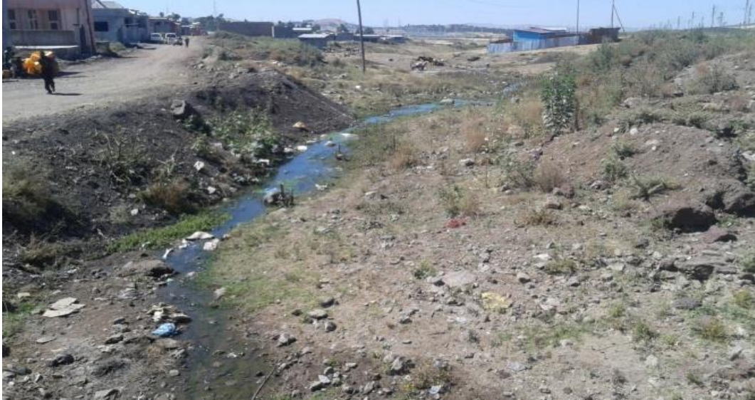
Figure 1.1: Existing polluted surface water in Gelan town
