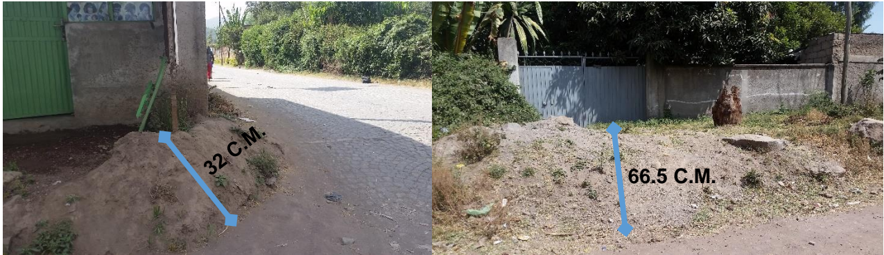
Figure 57. Soil Compacted Entrances
