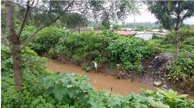
Figure 39. Non-Paved Drainage line serving as Waterway during Rainy Season
