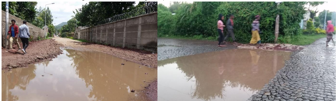
Figure 15. Lack Drainage line on the Street (Source: Field Photograph, 2017.)
