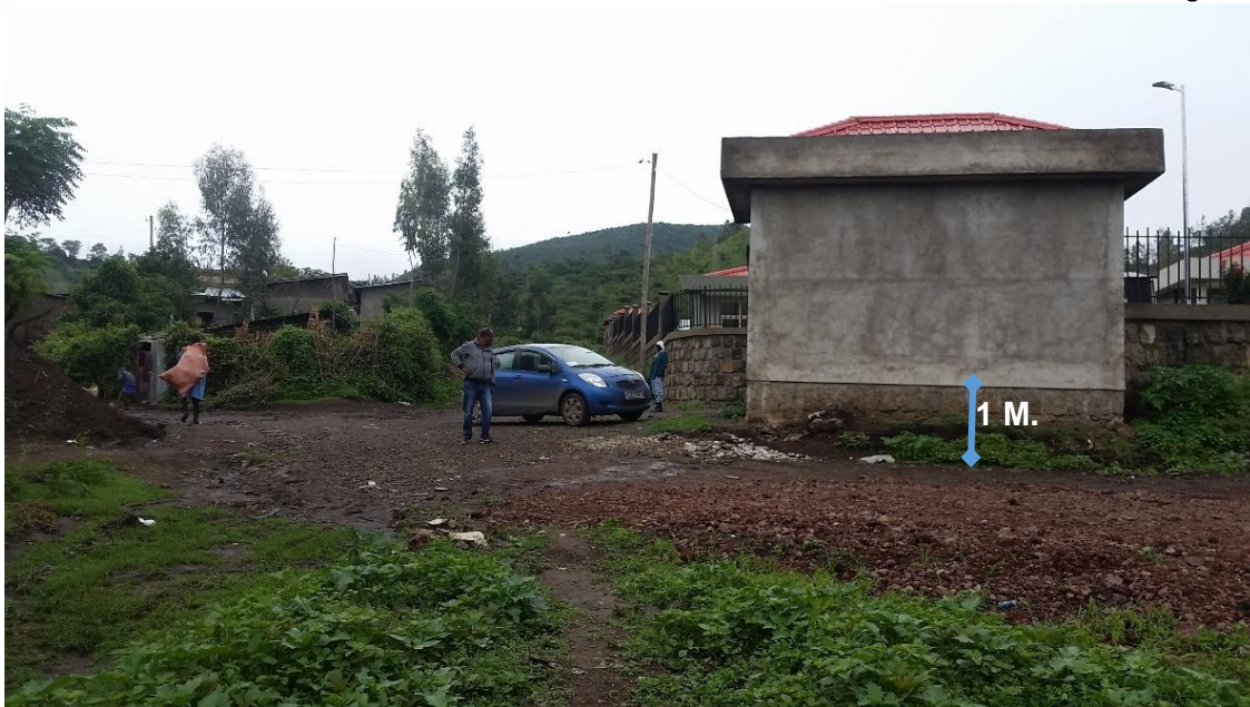
Figure 58. Housing Unit Foundations up to 1 M.
