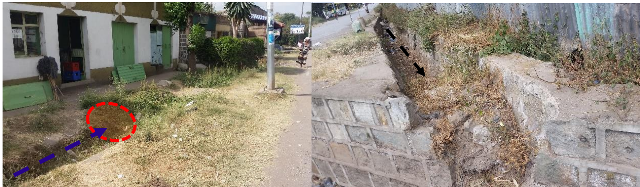
Figure 17. Dead end Drainage Lines
