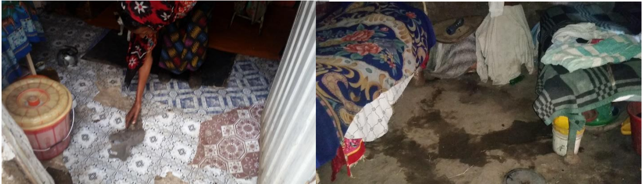
Figure 26. Housing Unit Floors Moistened from the Flooding (Source: Field Photograph, 2017)
