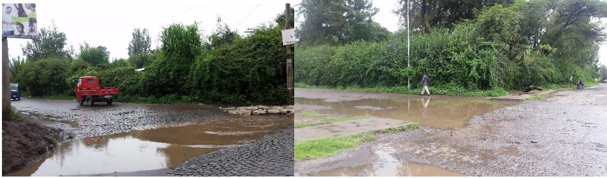
Figure 37. Poorly Constructed Cobble stone Paved Streets Promoting Inundation of Rain Water. (Source: Field Photograph, 2017)
