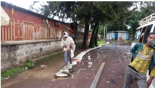
Figure 53. Sand Bags used as Walkway in swampy areas
