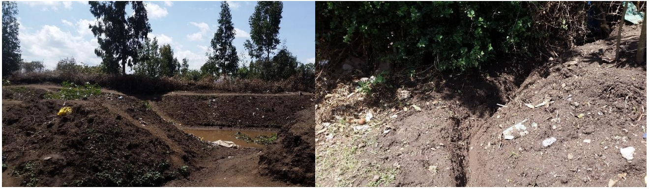
Figure 55. Diverging Waterway Strategy (Source: Field Photograph, 2017)
