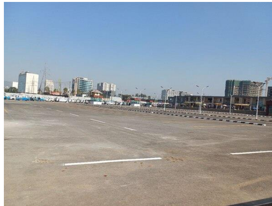
Figure 4.19: Parcel with Land Use Violation in Cherkos District (Mixed commerce to Surface Parking)
