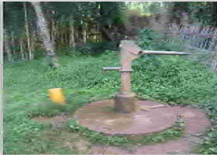
Figure 5.19 Hand dug well exposed for contamination in kale kebele
