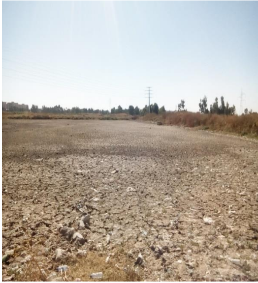
Sewage sludge in drying bed
