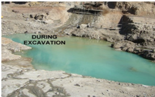
Plate 4.1 Artesian groundwater at the dam site
