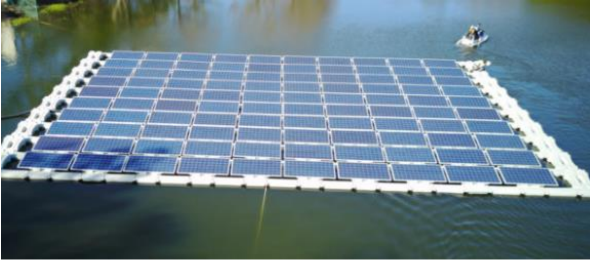
Figure 2. 4 Floating solar photovoltaic system (Jiang et al., 2023)
