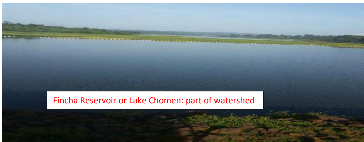
Figure 3.3 Upper Fincha Dam location
