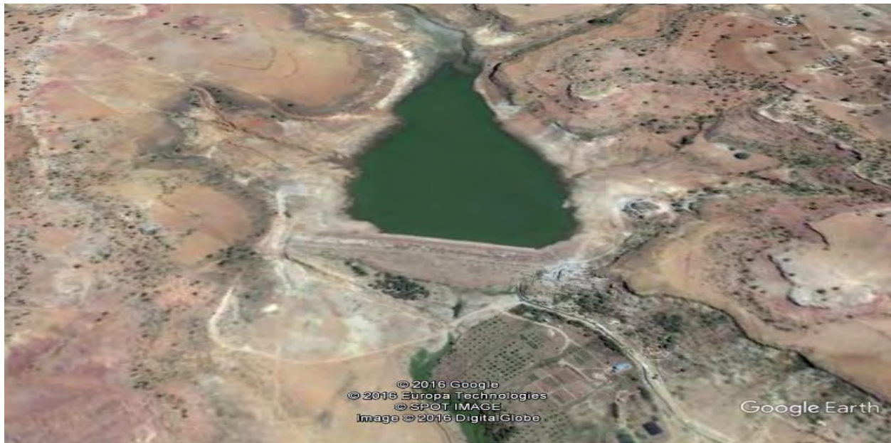
Figure 3.7 Location of Mygundi Reservoir Dam Site
