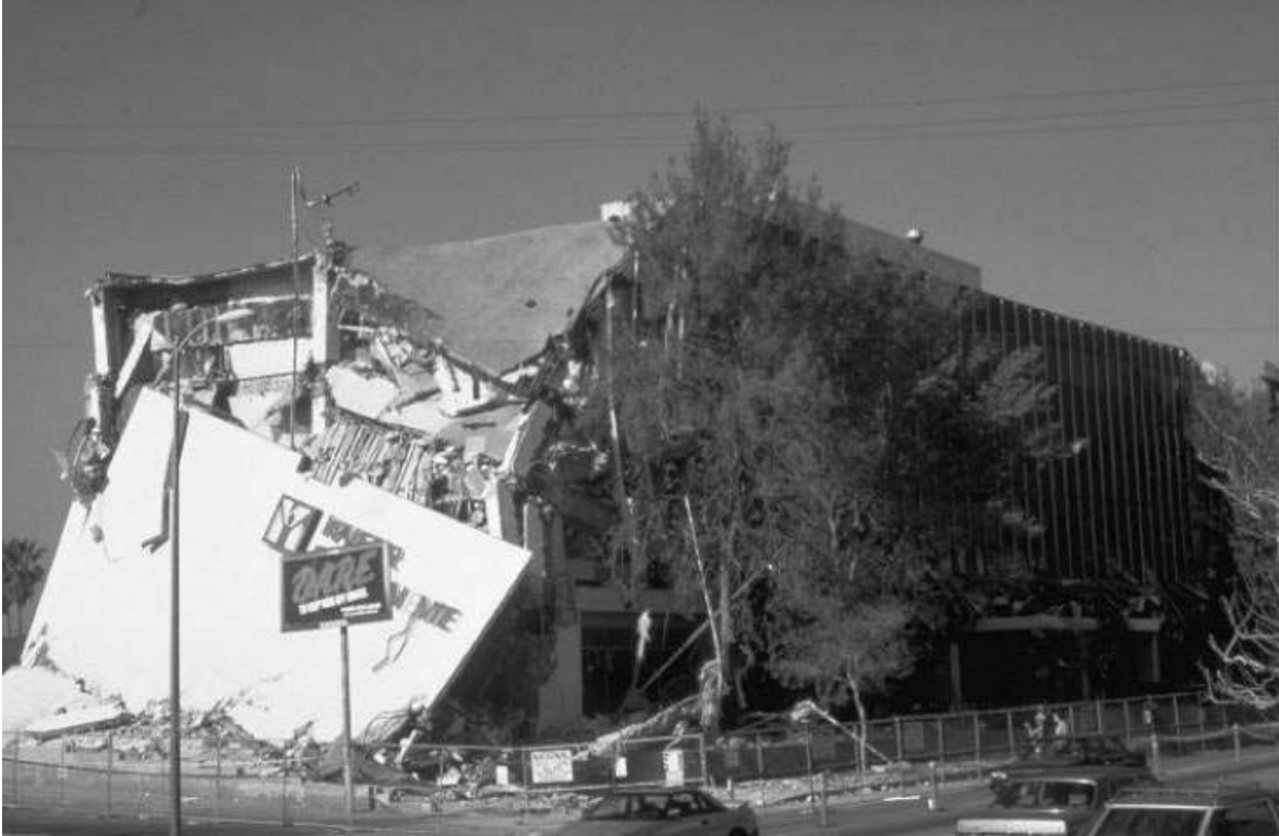
Figure 1-1 Collapsed end shear wall by Northridge earthquakes, 1994. Kaiser Permanente Office Building, Granada Hills, CA. (Photo courtesy of the University of California Library at Berkeley.)
