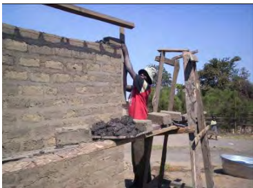
Fig.3.5 Housing being constructed
