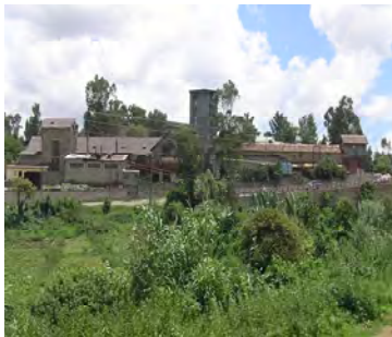
Fig.5.55 Mekanissa liquor factory
