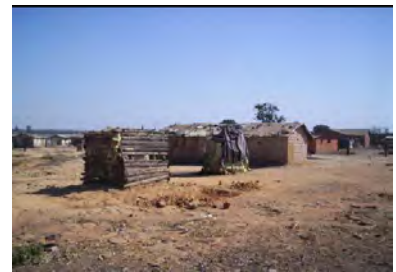
Fig.3.7 Timber & plastic covered pit latrines
