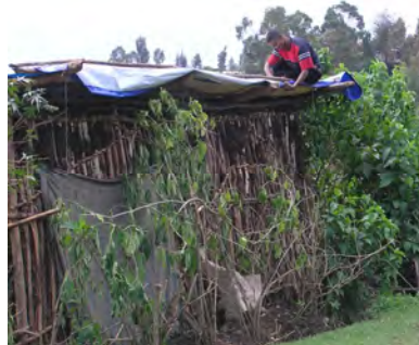
Fig.5.17- 2nd stage plastic roof cover
