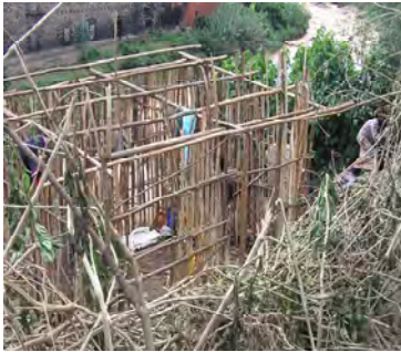
Fig.5.16- 1st stage wooden Wall erection
