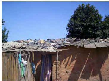
Fig.3.6 Roof made of various materials
