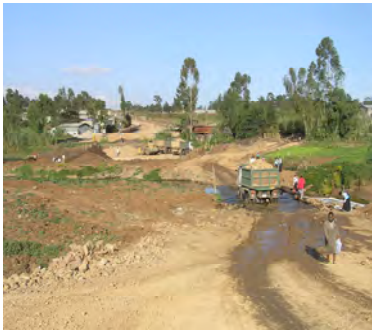
Fig.5.37 New road under Construction
