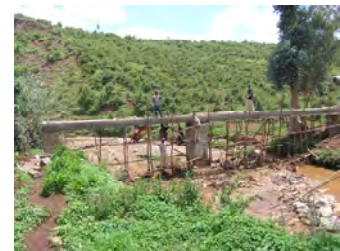
Fig.5.9 New concrete bridge
