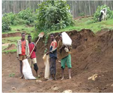
Fig.5.29 Red soil excavation For home use
