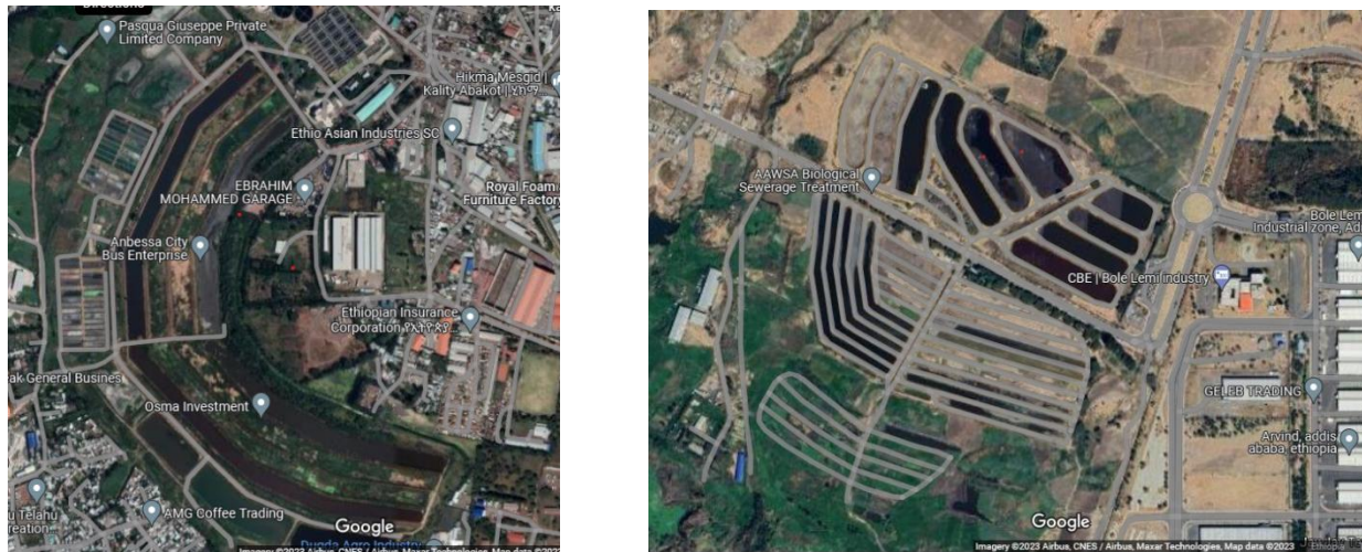
Figure 0.25: Addis Ababa city admiration water treatment plant (google satellite image)
