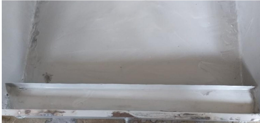
Figure 3. 6 : Condensate channel
