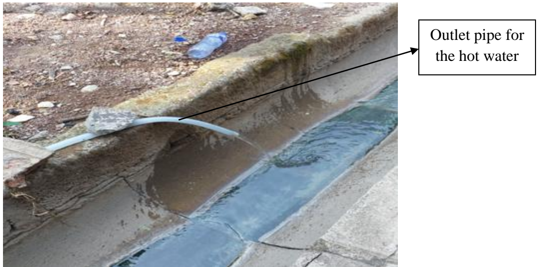
Figure 3. 18: The out flowing hot water from the geothermal still
