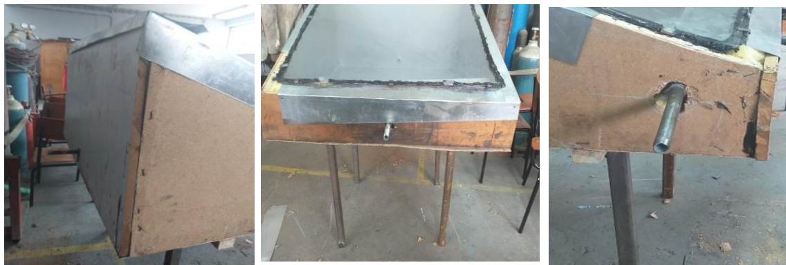
(a) Inlet pipe
