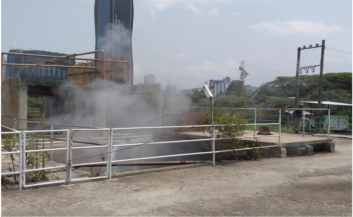
Figure 1. 1 : The collection chamber at the Finfine compound
