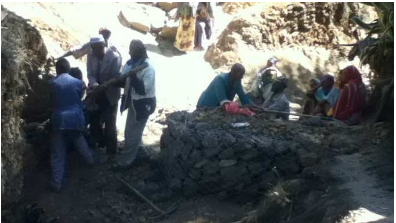
Figure 7: show that construction check dam by farmers.
