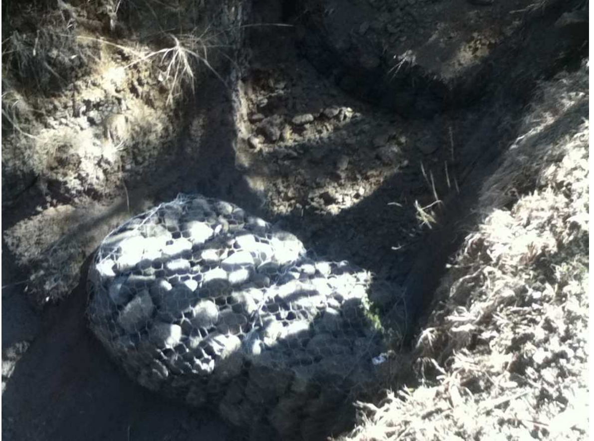
Figure 8 check dam made by stone and soil.
