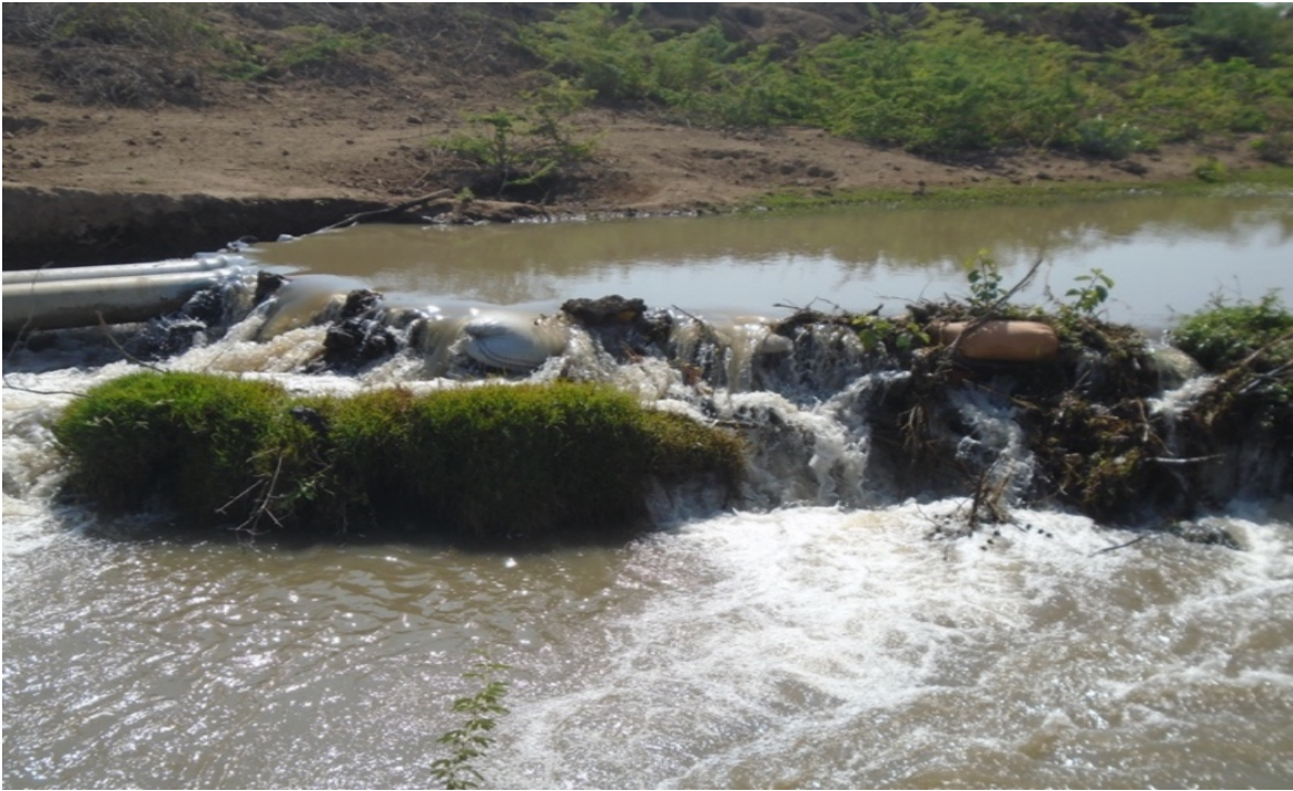
Photo 4: The irrigation canal blockage and water diversion at Xuxuxi and Ilaala (from top to bottom)
