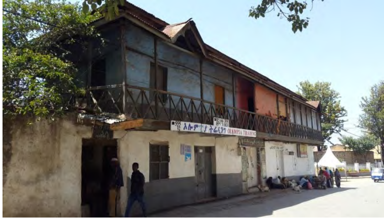
Figure. -3. Mahdi Adous's house (on the straight of Jegula Hospital), an example of traditional houses
