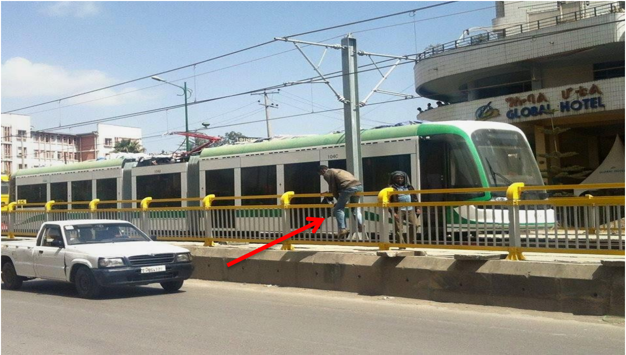
Figure 1: Pedestrians attempting to cross the newly built tracks with difficulty.
