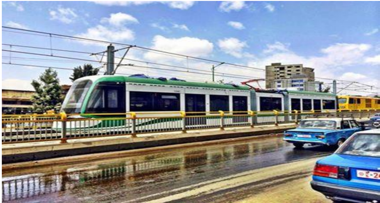
Figure 11: the Testing of Addis Ababa Light Rail Transit
