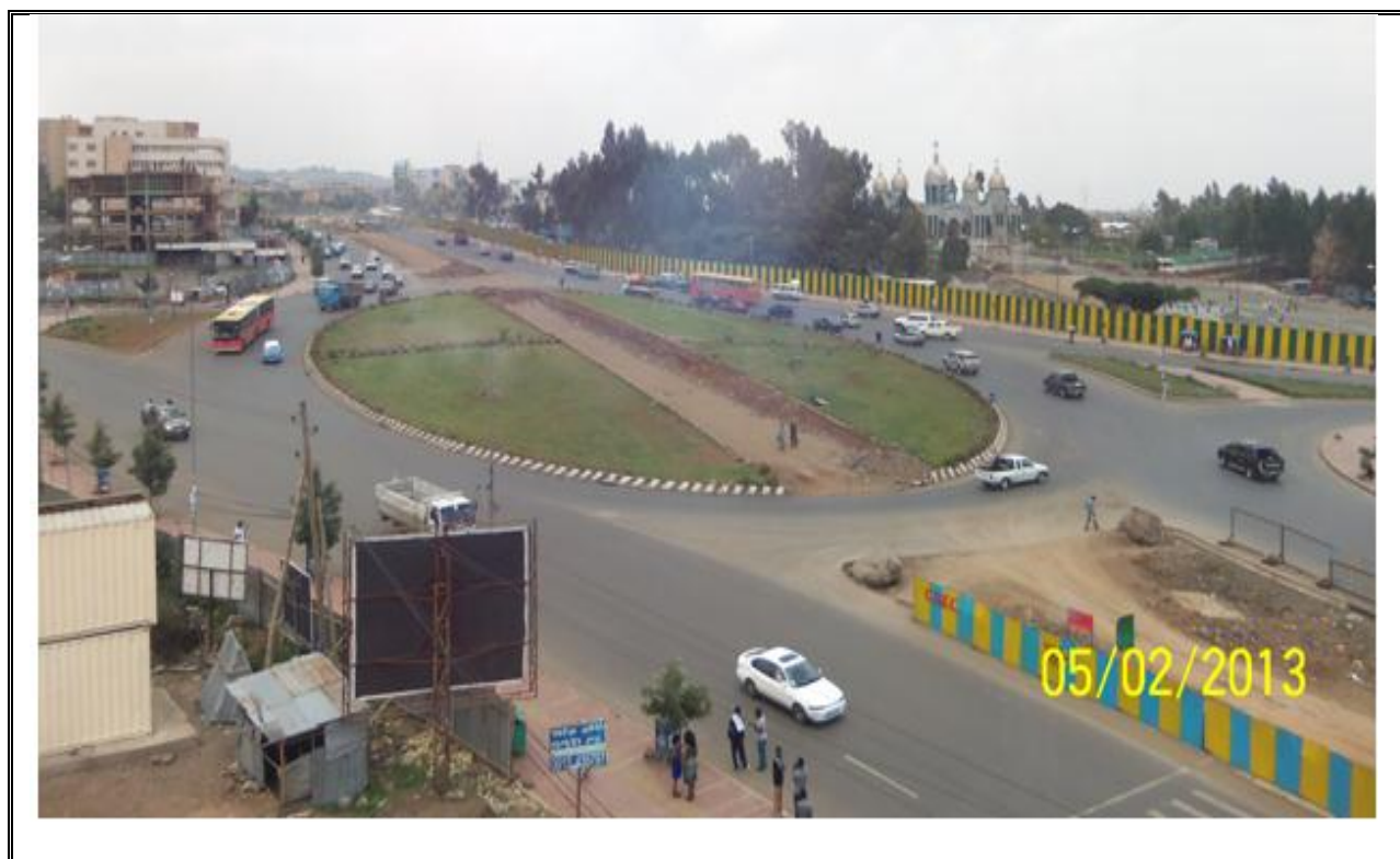
Figure 4-2 Top view of Beshale Hotel Round about Junction where the LRT crosses at-grade
