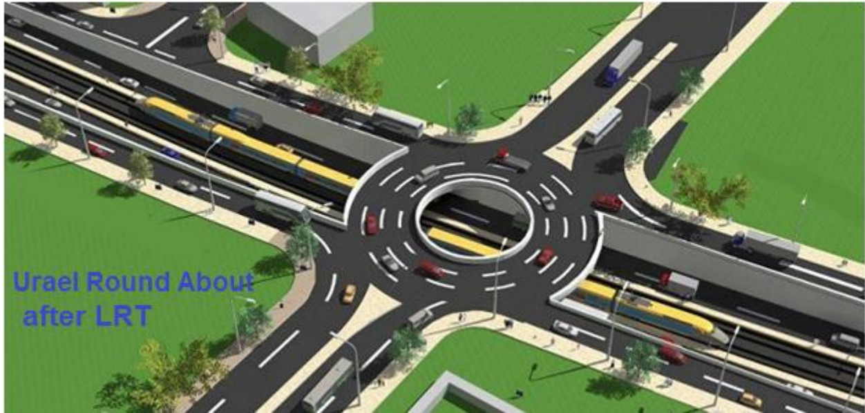
Figure 4-1 LRT grade separated at Mexico and Urael Round-About (Source: CORE Consulting Engineers PLC).
