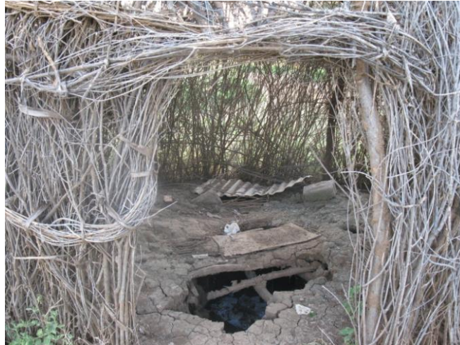
Figure 04: A Dangerous Dry Pit Latrine at Lokerlum Primary School in Nyangatom Woreda
