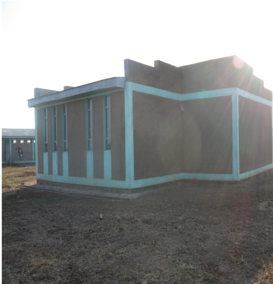
Figure 06: One of the Standard Blocks at Kibish Primary School, Nyangatom Woreda
