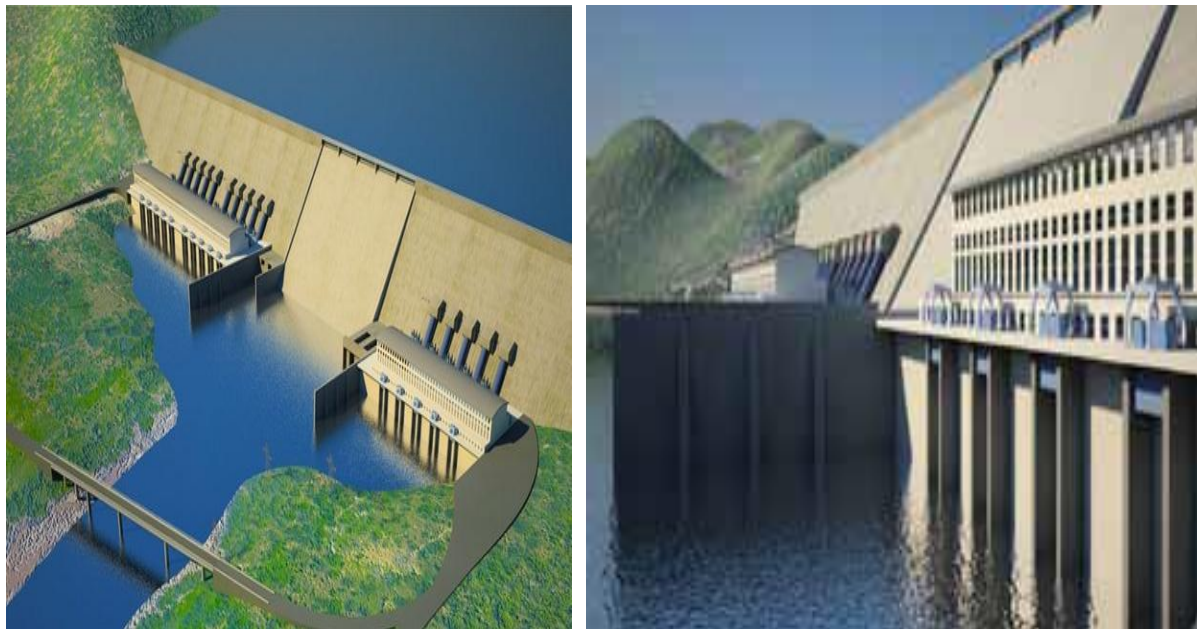
Figure 4.1: Artist's impression of the Renaissance Dam, under construction on the Blue Nile Source: MoFA, 2012 available at www.foreignaffairs.com/ethiopia-sponsored-section .
