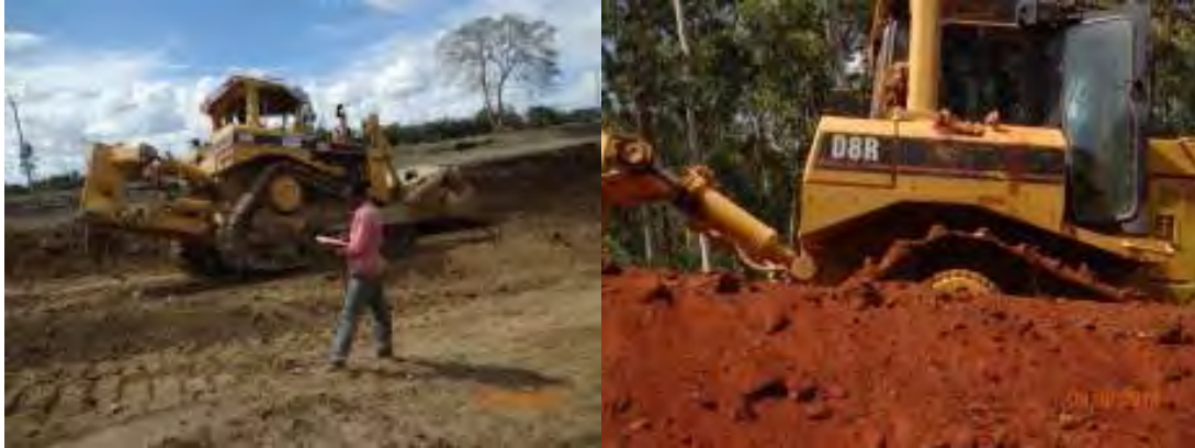
Excavating and pushing earth material using dozer
