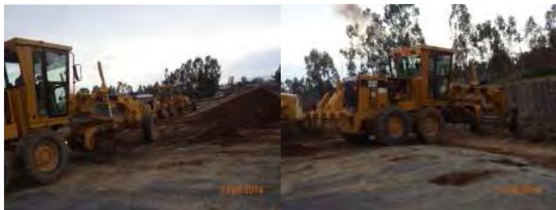
Spreading and leveling of sub-base material using motor grader
