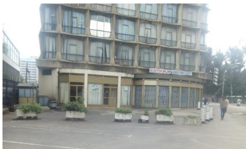
Figure 64: Outdoor open area
