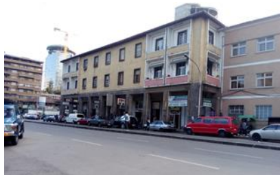
Figure 17: Lower level view
