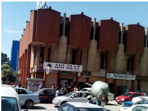
Figure 86: Lower level view
