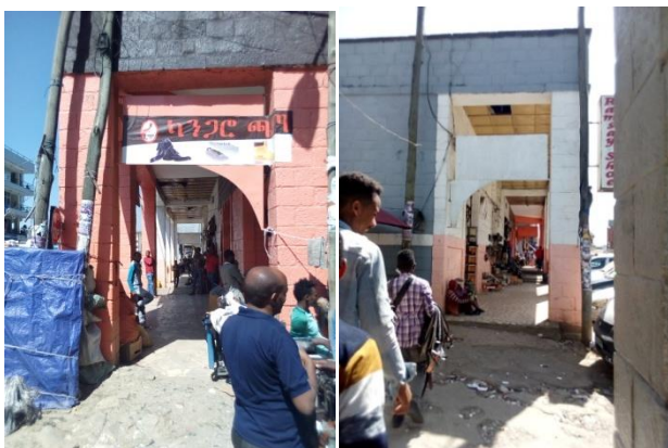
Figure 72: Lower level view
