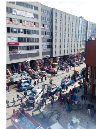
Case study building/Mars Commercial center
