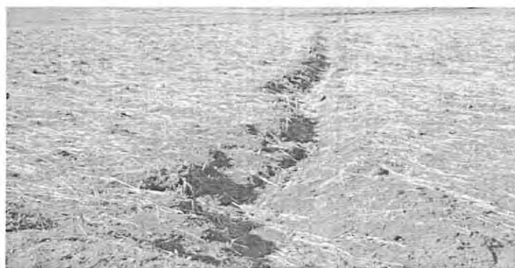
Picture3. Erosion Risk of Widening Ditch at the End Point Photograph taken by the author, 2009
